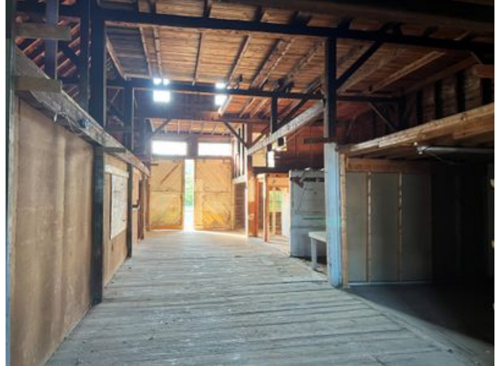
Barn First Floor Interior
