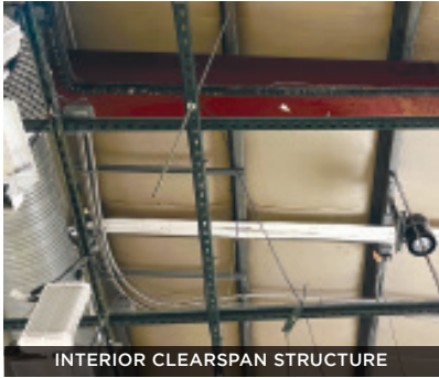
INTERIOR CLEARSPAN STRUCTURE
